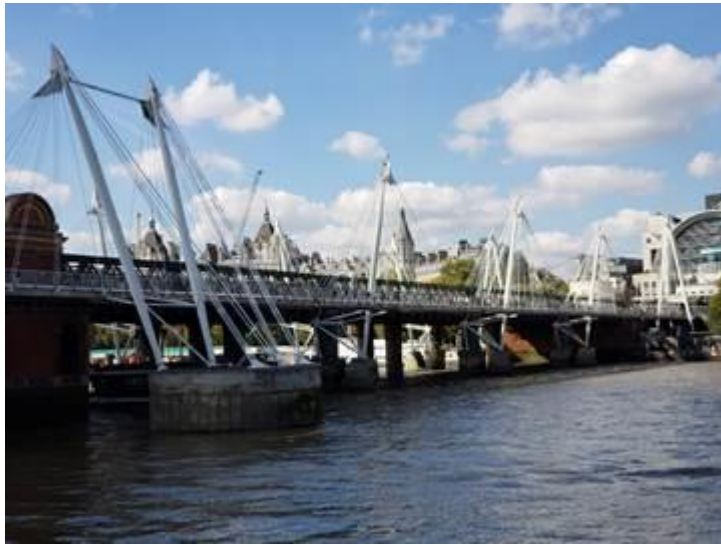
Hungerford Bridge and Golden Jubilee Bridges Construction: 1859 and 1996 Opened: 1864 and 2002 Clearance Below: 34' Length: 820'
