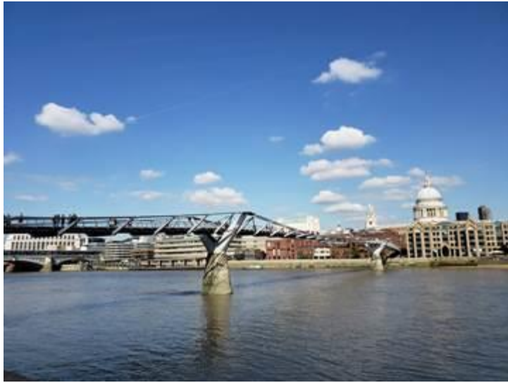
Millennium Bridge Construction: 1996 Opened: 2000 Clearance Below: 35' Length: 1,066'
