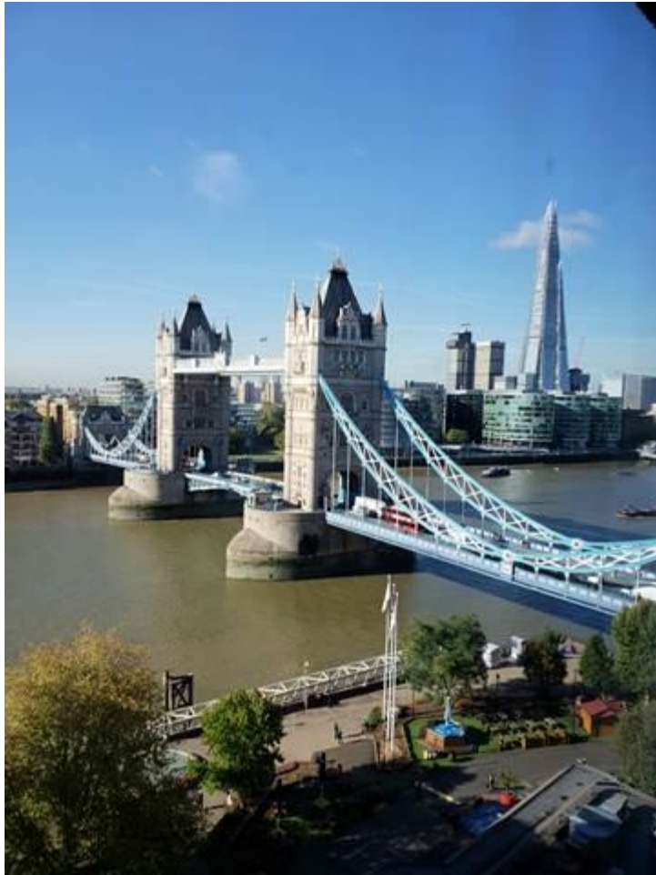
Tower Bridge Construction: 1886 Opened: 1894 Clearance Below: 28' Length: 801'
