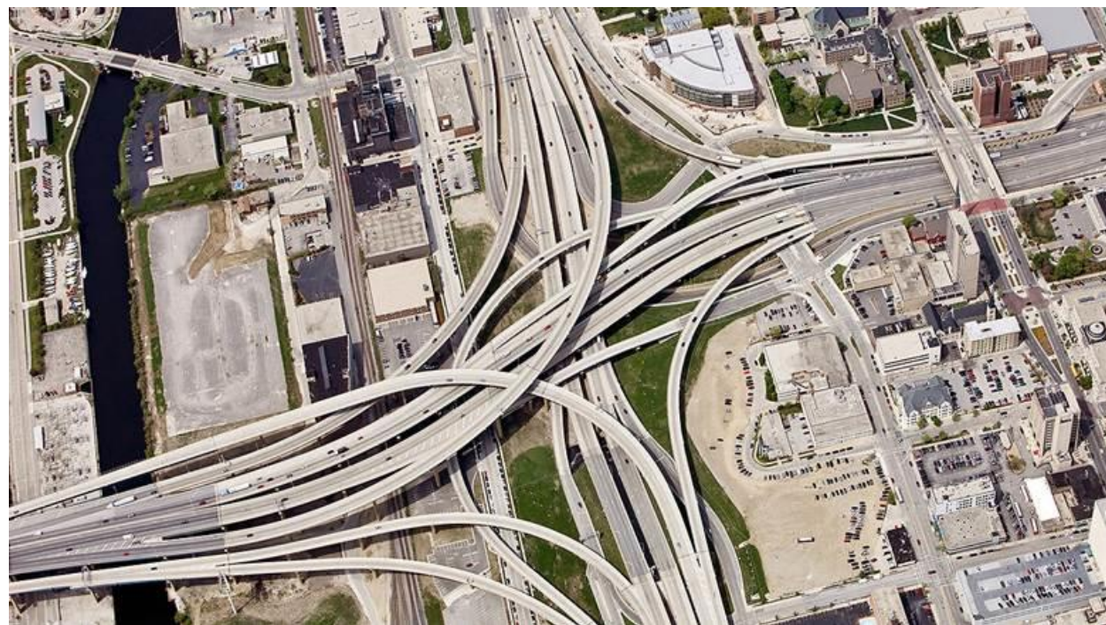
Overhead highway view
