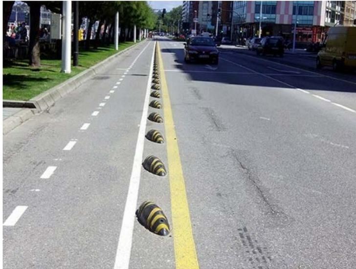
UK-based [Cyclehoop](#) has found a way to use pieces of recycled plastic to keep [cyclists](#) safe on the road. Their clever "Armadillo" lane dividers can be easily installed on roads to divide bike lanes from traffic and gently remind cars to steer clear of cyclists. The affordable solution could significantly help improve [road safety](#) and reduce accident
