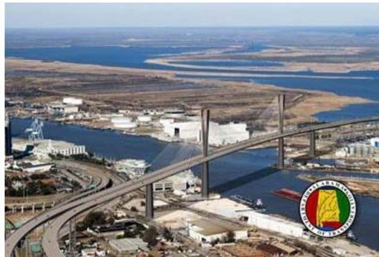
The I-10 Mobile River Bridge and Bayway Widening project is a proposal to increase the capacity of I-10 by constructing a new six-lane bridge with 215 feet of Air Draft Clearance (ADC) across the Mobile River and widening the existing I-10 bridges across Mobile Bay from four to eight lanes. The proposed project would be located in Mobile and Baldwin Counties, Alabama.
